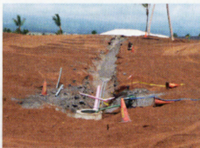
A PVC liner (left photo) goes down before drain tile (center photo), "choker" layer and greens mix are installed (details in illustration below). Drainage from holes 12 through 17 goes to wet wells (right photo) before being pumped to inland dry wells.
