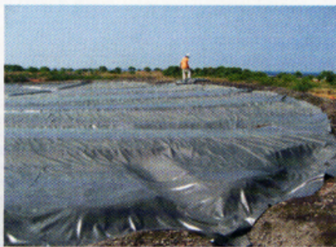
A PVC liner (left photo) goes down before drain tile (center photo), "choker" layer and greens mix are installed (details in illustration below). Drainage from holes 12 through 17 goes to wet wells (right photo) before being pumped to inland dry wells.
